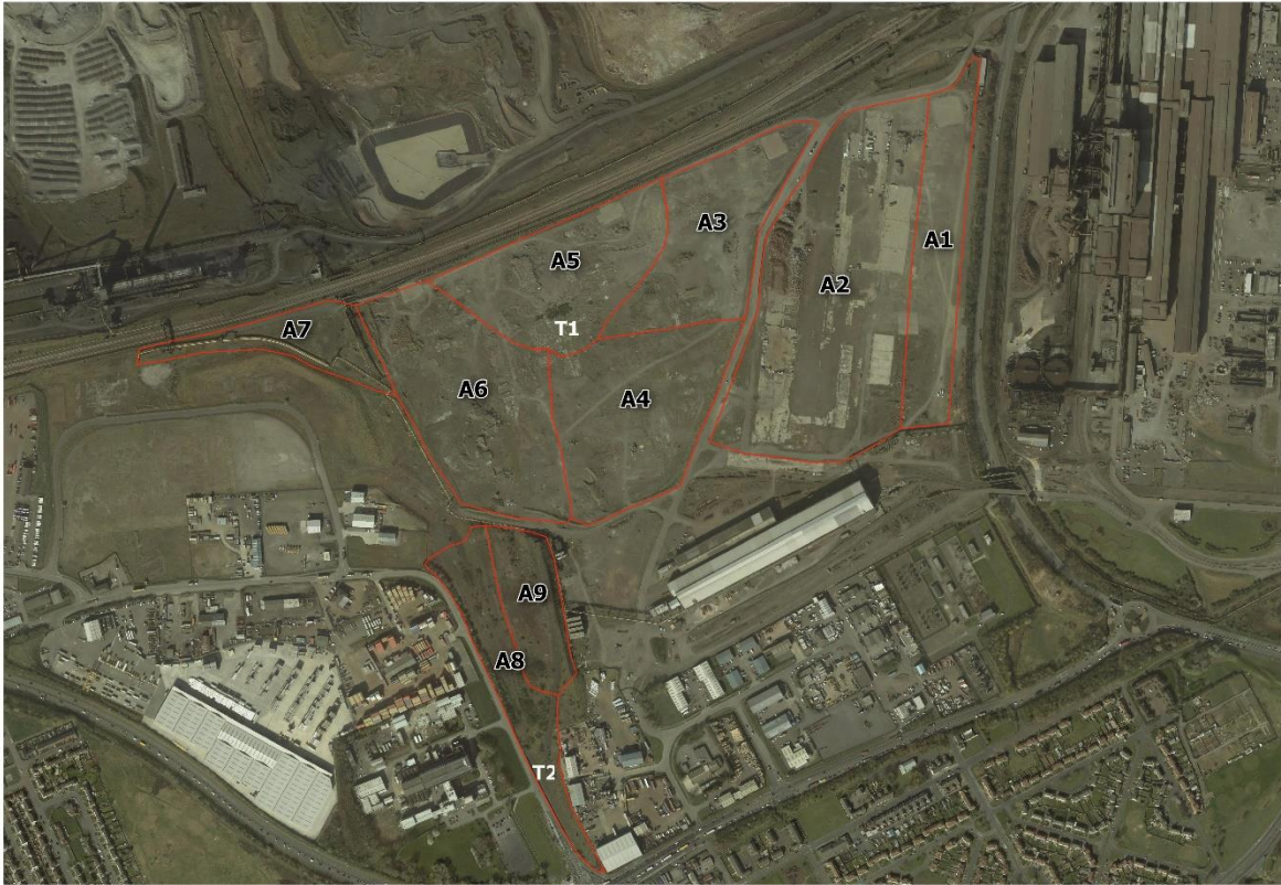
Figure 3. Broad areas of vegetation types (Target notes are shown as T1 and T2) Cross-reference to INCA (2018)
